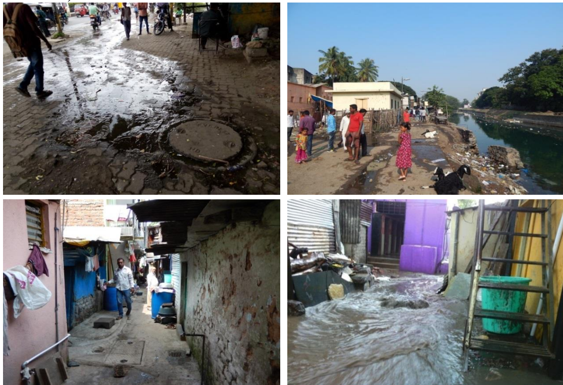
Figure 5.15: Basic Urban Service in Pune – Drainage: (i) Gosavi Vasti; (ii) Panmala; (iii) Wadarvadi; and (iv) Flooding at Saibaba Vadarvasti last year (From top left clockwise)
